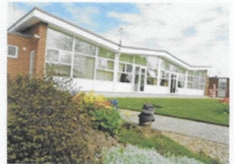
Southfield House, Woolram Wygate
